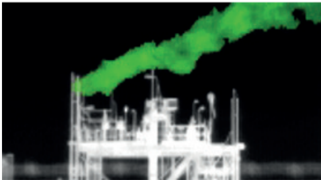
Freon 22 detected from a 350-m distance in real time and quantified with the Hyper-Cam. Calculated leak rate was determined to be 10 000 g/h.
